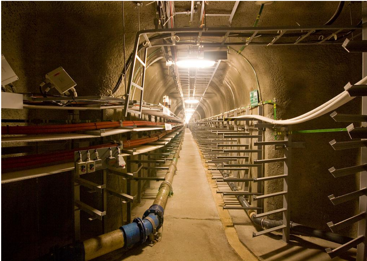
Tunnel in Prague is shared by pipes and cables
